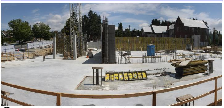
Onstruction of the new school has passed a significant milestone with the pour of the main floor in June. *Mr. Horton's* photograph this month was taken from Room 504 in the Science Wing looking east and shows the main floor in place and shoring for the gymnasium walls going up.
